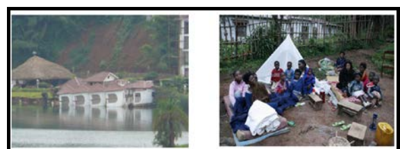
Fig.12: Landslides and loss of houses because of earthquake in February 8, 2008
